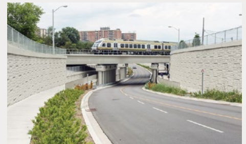
DENISON ROAD GRADE SEPARATION
