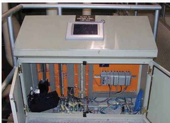
Filter control panel post-commissioning, in which, the new controller and HMI interface panel have replaced the legacy system highlighting a much “cleaner” installation.
