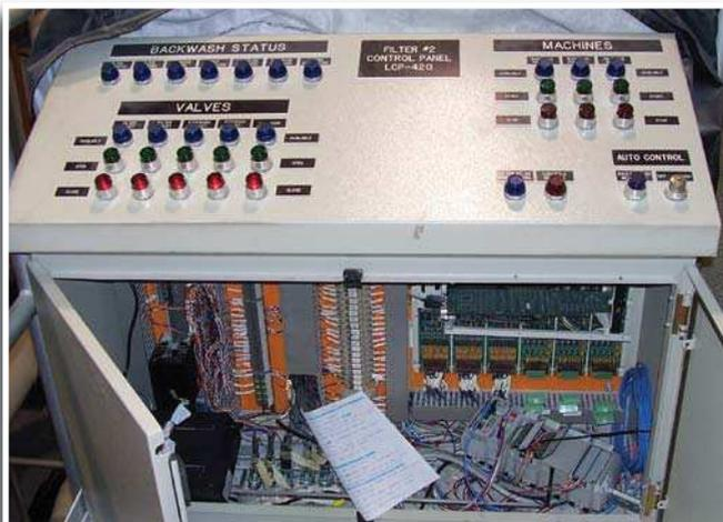
Filter control panel depicting the legacy and new PLC controllers on the same I/O set.
