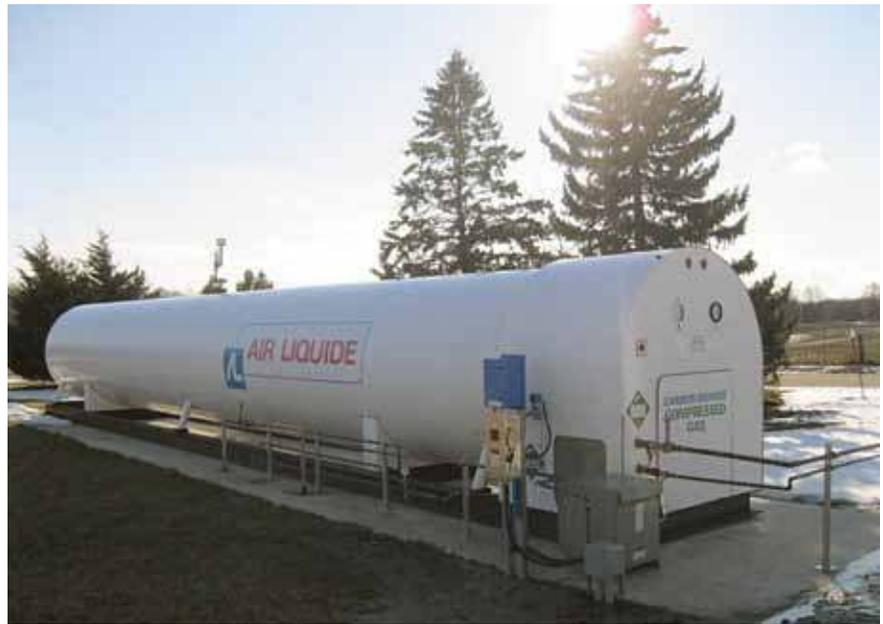
Figure 3 – Carbon Dioxide Storage Tanks
