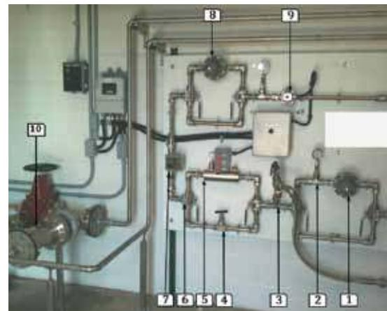
**Figure 1 - Carbon Dioxide Chemical Metering Panel**
