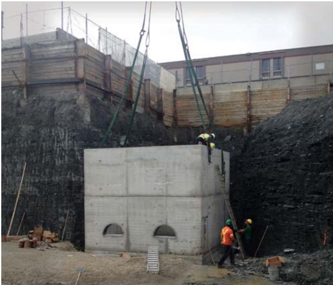
Custom Made Precast Concrete Stormwater Detention System
