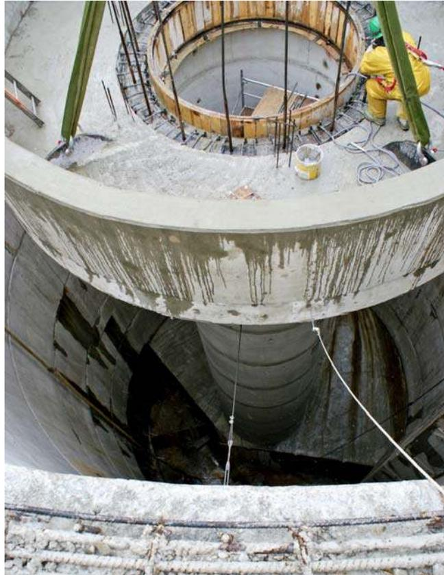
Figure 6. Photo of the assembled overflow structure.
